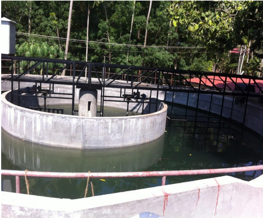
Treatment Plant: Clarifier Work in Progress
