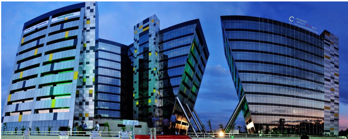
View of IT Building in Technopark Phase III
