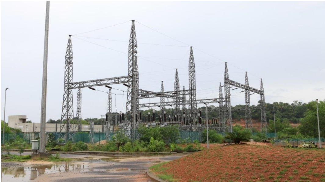
Work progress of 110 kv Substation.
